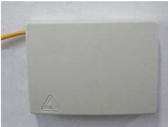
Pic22: cover the terminal box
