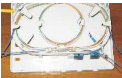
Pic14: after shrink, splice protective tube put into the slot
