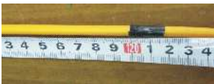
Pic 3:the length of stripped fiber cable Pic4: fiber after stripping Pic5: use EVA transparent tube to protect the stripped fiber
