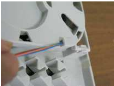
Pic9: thread the fiber to the cable inlet
