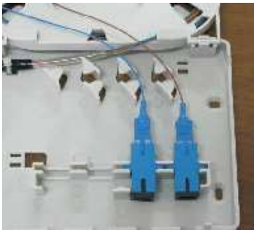
Pic11: install the adaptor and pigtail
