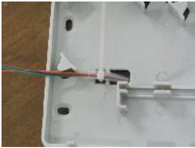
Pic6: dark-routing leads in box fixes by nylon tie
