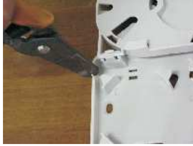
Pic7: right-routing leads in box entrance and fixes by nylon tie
